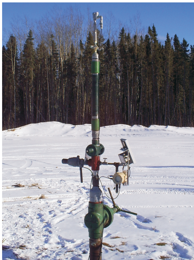
Northern Canada installation monitoring both surface as well as downhole pressure
