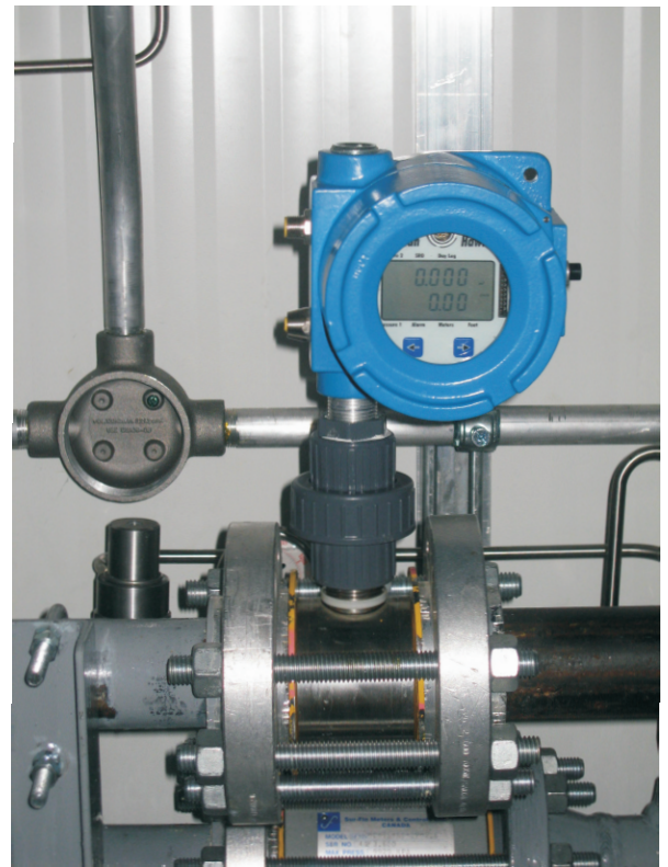
Hawk 9500 IS Model Field Install
