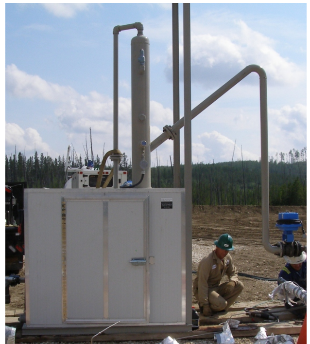
Northern Alberta Installation June 2006
