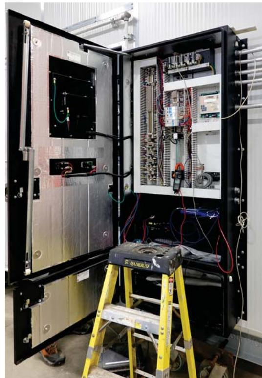
A separator control panel undergoing a power audit. The bottom part of this cabinet is inserted in the separator building and holds eight AGM batteries.
