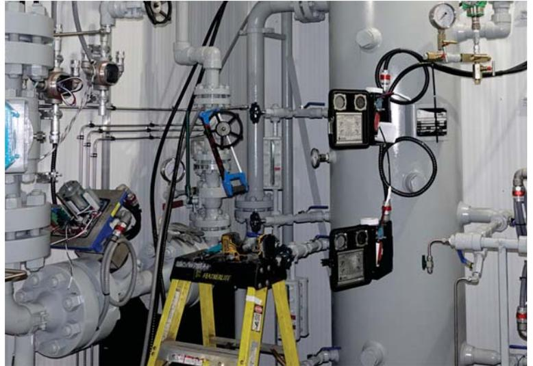
A 3 inch BTE Forum Choke outfitted with a Bear LA-7 Electric ¼ turn actuator and electric level controllers being installed
