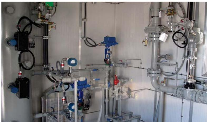
Two fast acting Bear SA linear actuators used on Fisher D2 dump valves and on the right a BA-15L being used for outlet back pressure control
